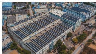
1.4MW - MTAR, Hyderabad
